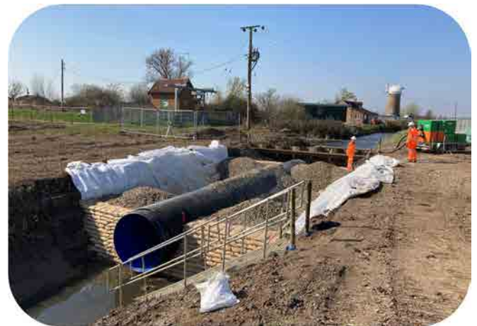
Above: Construction of the new access culvert at Potter Heigham replacing the existing failing corrugated steel culvert
