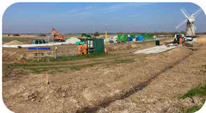
Above: Site set-up and mitigation complete at St Benets pumping station. UK Power Networks shown disconnecting the existing power supply.
