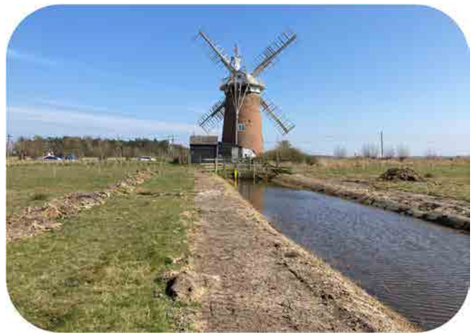
Above: Watervole mitigation works completed at Horsey pumping station at the location of the new pumping station inlet
