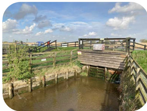
Stracey Inlet from River Yare discharges into Stracey Mill outlet channel
