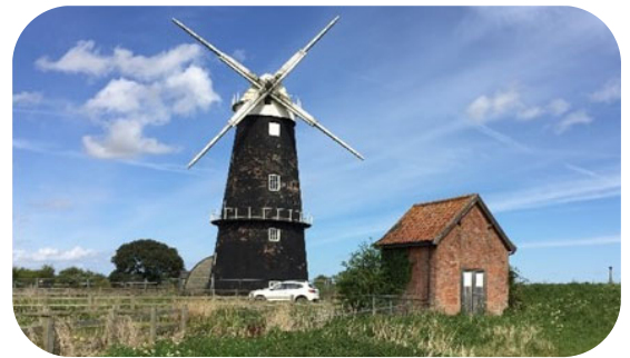
Berney Arms Pumping Station
