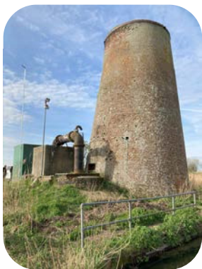
Buckenham Pumping Station
