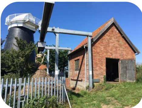
Norton Pumping Station
