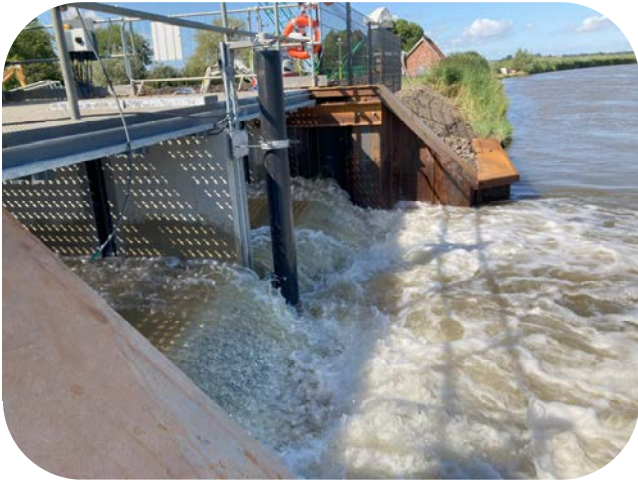
The Outfall, during the wet testing of the new pumps.
