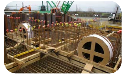
Concrete forming for pumping stations inner workings. Photo credit BAM UK
