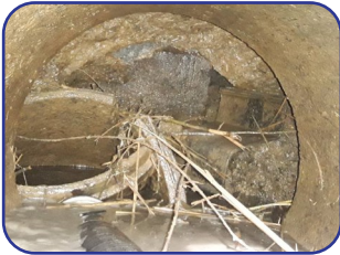
Culvert beneath Barsham Brook
